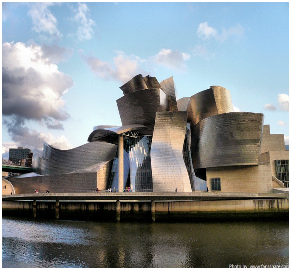
Gehry's Guggenheim Museum in Bilbao, Spain: photo credit Fanshare
